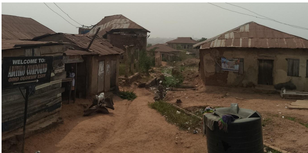
Figure 2. Drainage Condition in Isale-Osi Area Source: Authors' Field Work, 2026.
